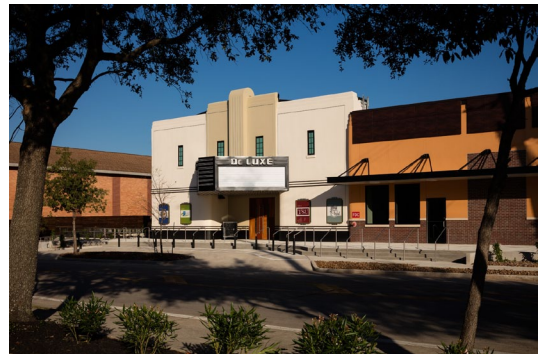
Photos: Left, groundbreaking ceremony; Above, a shell of a building; ribbon cutting on new theater 2015; new streetscape (photos courtesy Smith & Company Architects)
